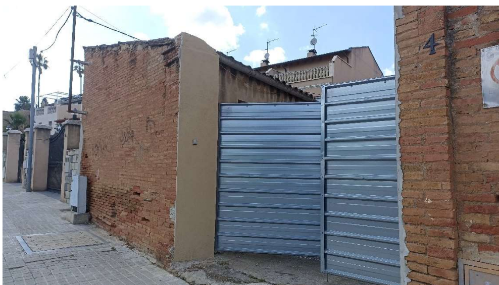
porta provisional existent (exterior)
