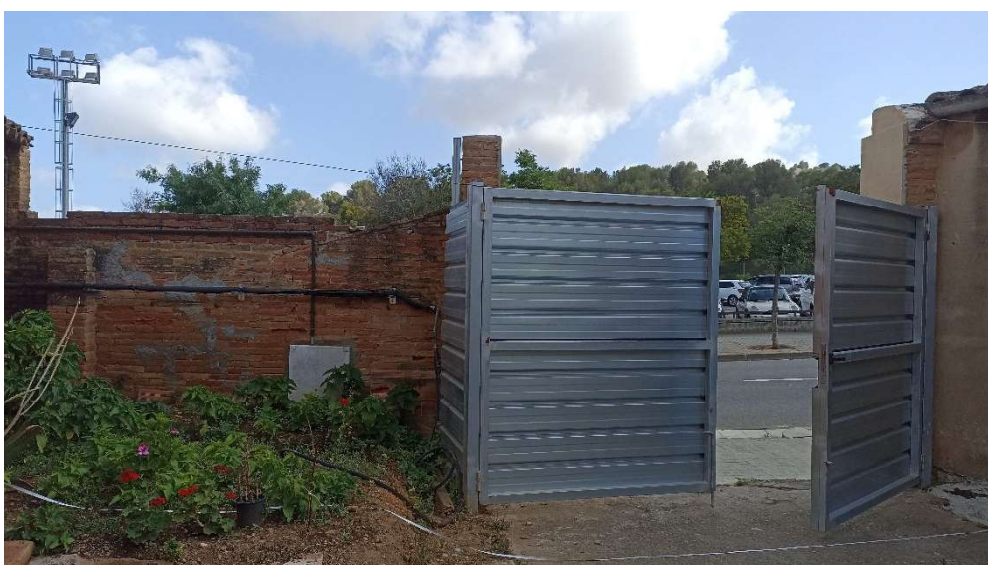
porta provisional existent (interior)
